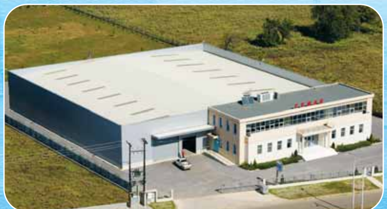
Premises 2.600m 2 THESSALONIKI - NORTH GREECE
