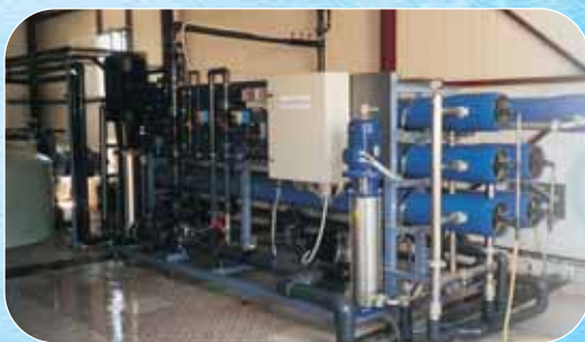
HOTEL PORTO HYDRA/GREECE
